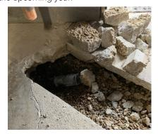
Skyview were leaking. One was located under the cement which required removal to access.
